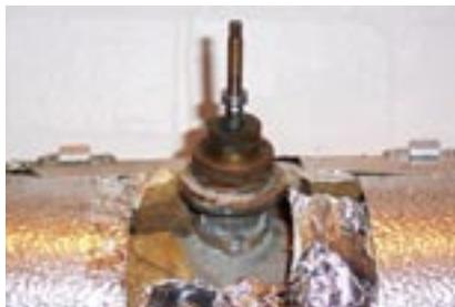
The linkages used within the British Library for mounting the Belimo actuators were the Belimo UNV-023 (Satchwell) and the UNV-025 (Osby). The simple fitting concept shown below is the same for all of the Belimo linkages.
